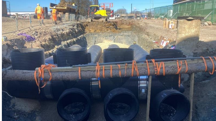
Attenuation Pipework in progress West
