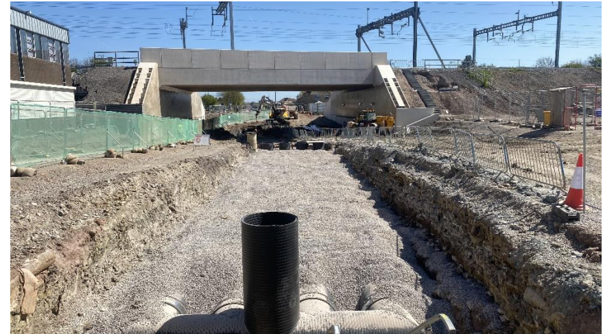
Attenuation pipework complete at West end progressing under bridge
