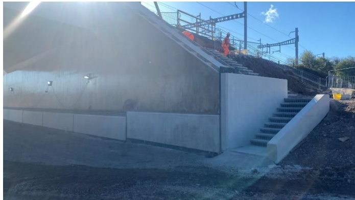
South West Wingwall complete and Steps in progress
