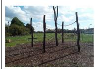
I have also highlighted my main concerns with the equipment as it stands, aiming at the rotten timber beams at ground level causing too much movement to the main structure. As we have a duty of care to the users and the fact the item of equipment is a main focal point to the park I feel we should look to replace the item asap, or remove the current climber during the autumn of 2023 due to its continued deterioration especially through the winter months.
